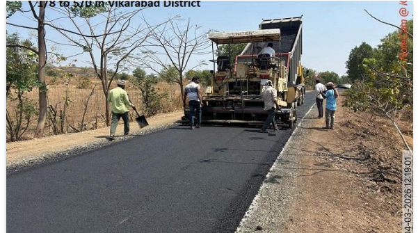
Periodical Renewal Work is in progress on Kesaram - Turumamidi road in Vikarabad Dist
