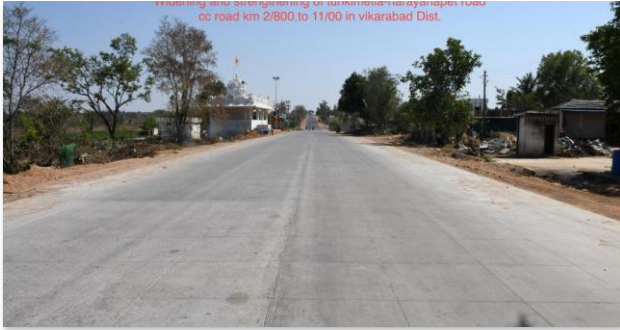
W & S of Tunkimetla - Narayanpet road in Vikarabad Dist.
