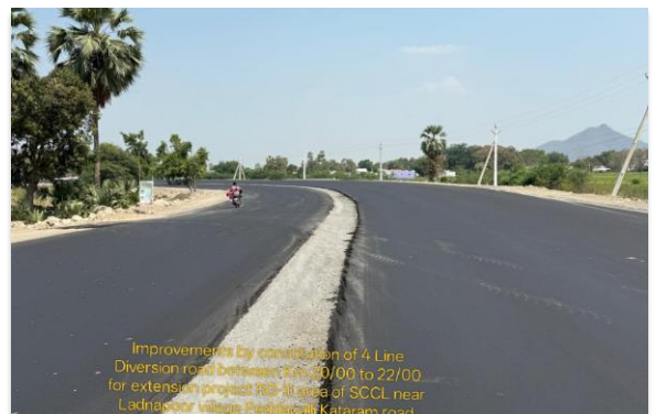
Improvements to Peddapalli - Kataram road in Peddapalli Dist.
