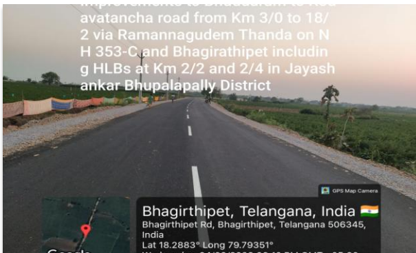
Imp to Bhuddavaram to Kodavatancha in JS Bhupalpally Dist.
