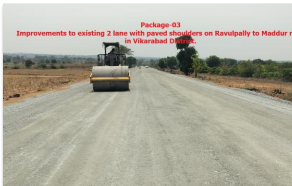
Imp to Ravulpally to Maddur road in Vikarabad Dist.
